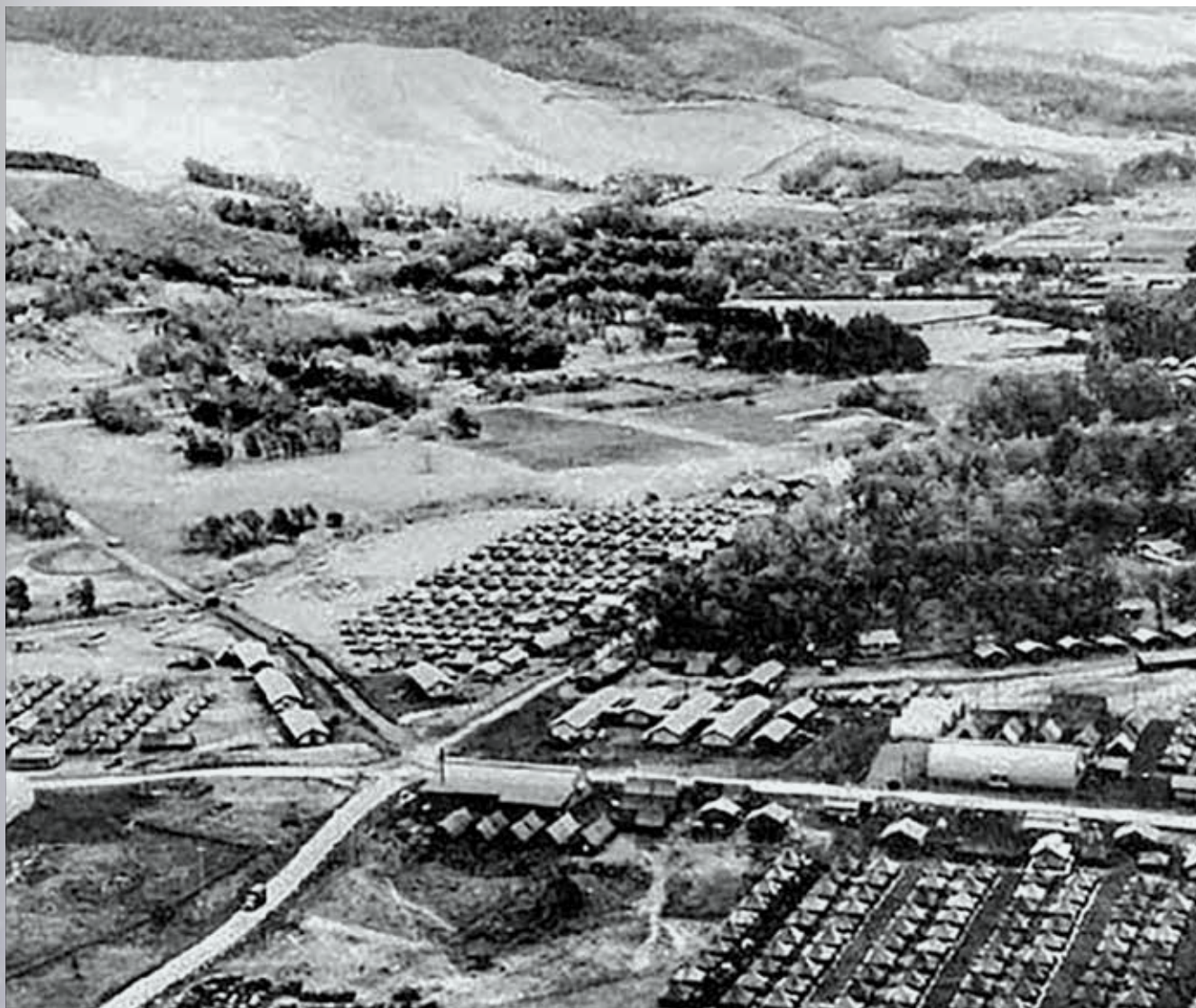
Aerial view of Camp Tarawa. When they think of Hawaii, most people think of palm trees and beautiful beaches, but that's not where they put Marine bases! Camp Tarawa was located between two volcanoes at a 2,670-ft elevation where it is very windy and cold at times.
